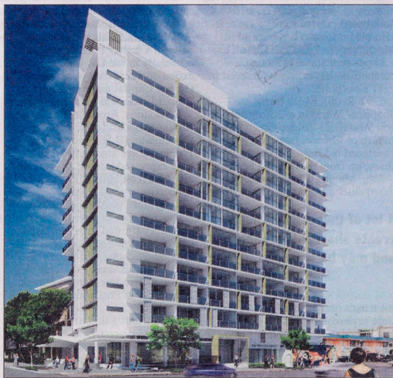
Artist's impression of Alex Perry apartments, which will be marketed this month.
